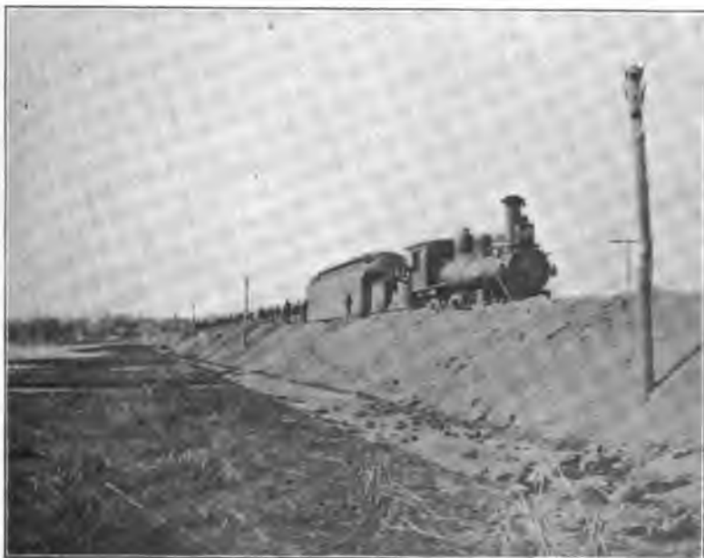
Mauricetown Bridge road, Cumberland Co., under construction ; fill across marshes.
